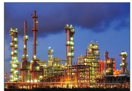
Oil and gas, chemical and petrochemical Plants
